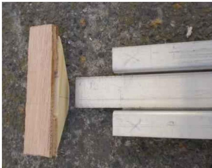
*Fig 8. Instead of a bolt as used in the unit above, bars now go into a wooden support mounted against the bulkhead. Seen here is the wooden fitting, bar and top-hat section.*
